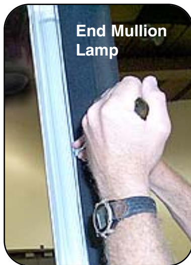
Figure 21. Removing Diffuser from End Mullion Lamp
